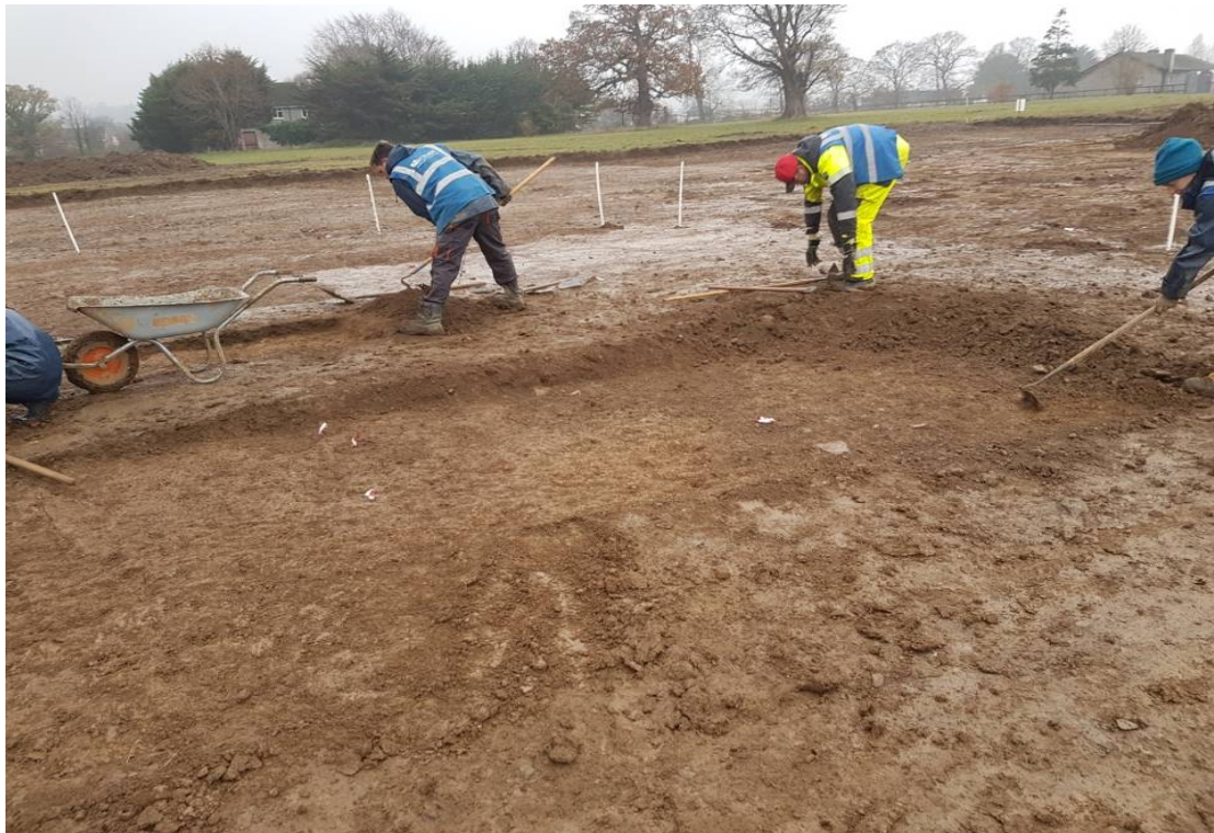
Plate 3: Hand removal of lower topsoil
