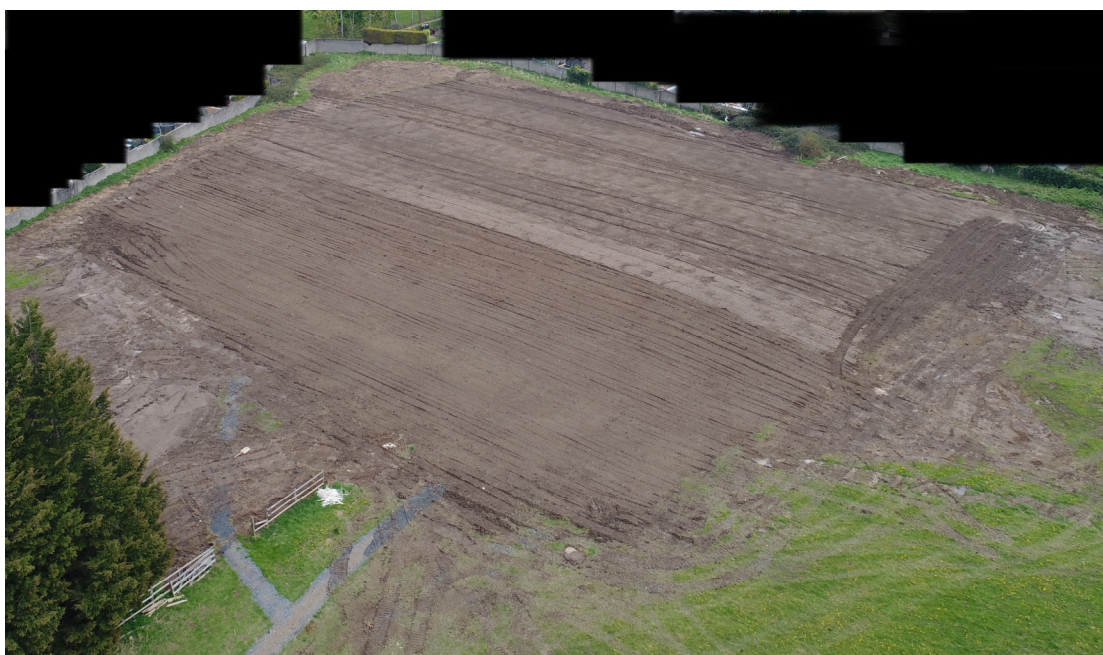
Plate 11: Aerial view of site following backfilling
