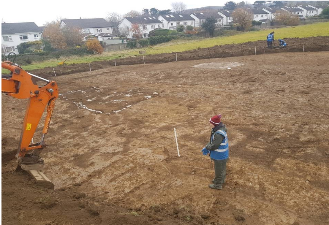
Plate 2: Topsoil stripping in foreground & metal detection in background
